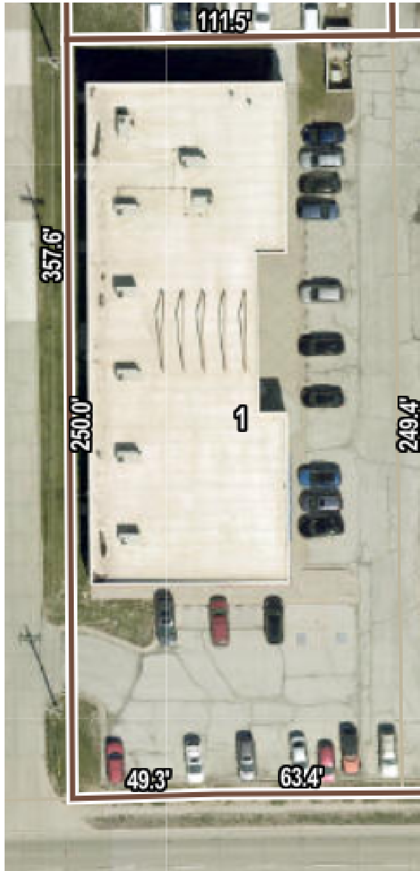
Hillcrest Health Offices - Building 1 1820 Hillcrest Drive
